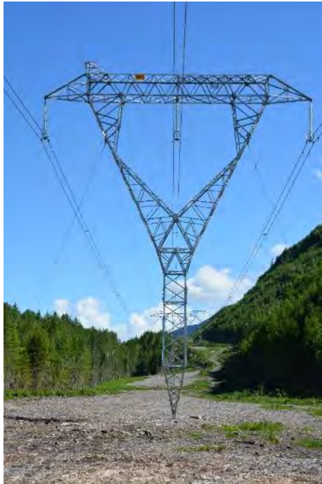
Figure 18-24: Typical 287 kV Guyed Tower
